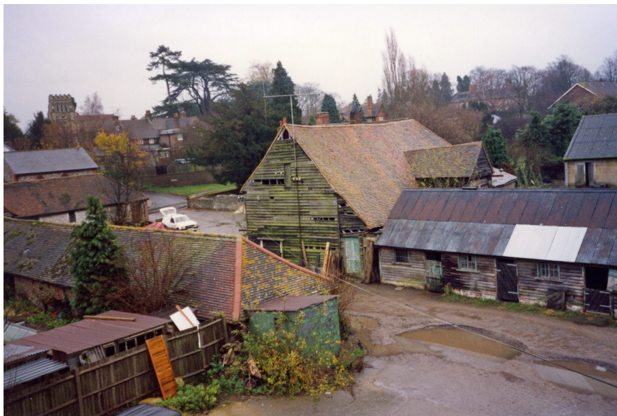
Figure 13 View of the west-facing side of Home Farm barn, early 1990s, before later repair and refurbishment.
