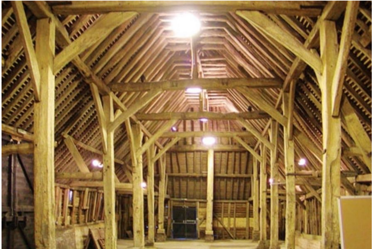
Figure 11 The interior of Wanborough Great Barn – not a tithe barn.
