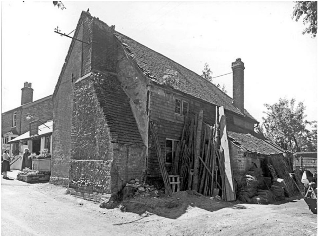
Figure 27 The poor state of Forge House as photographed by D Yellan on 2 June 1959.
