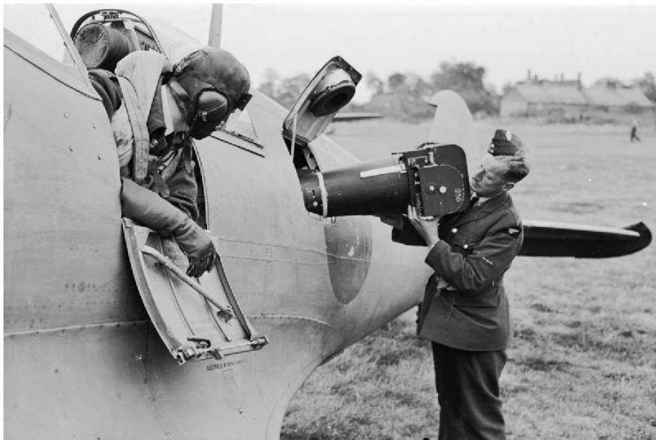
Figure 11 A Type F.8 Mark II (20-inch lens) aerial camera being loaded into the vertical position in a Supermarine Spitfire PR Mark IV at RAF Benson; Imperial War Museum Image IWM (CH 10847).
