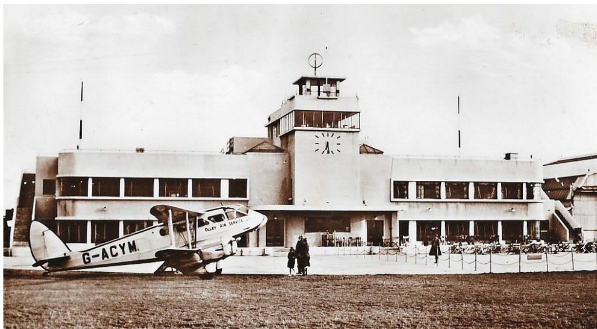
Figure 3 Terminal building at Shoreham-on-Sea, late 1930s; at left – a De Havilland DH.89 Dragon Rapide.
