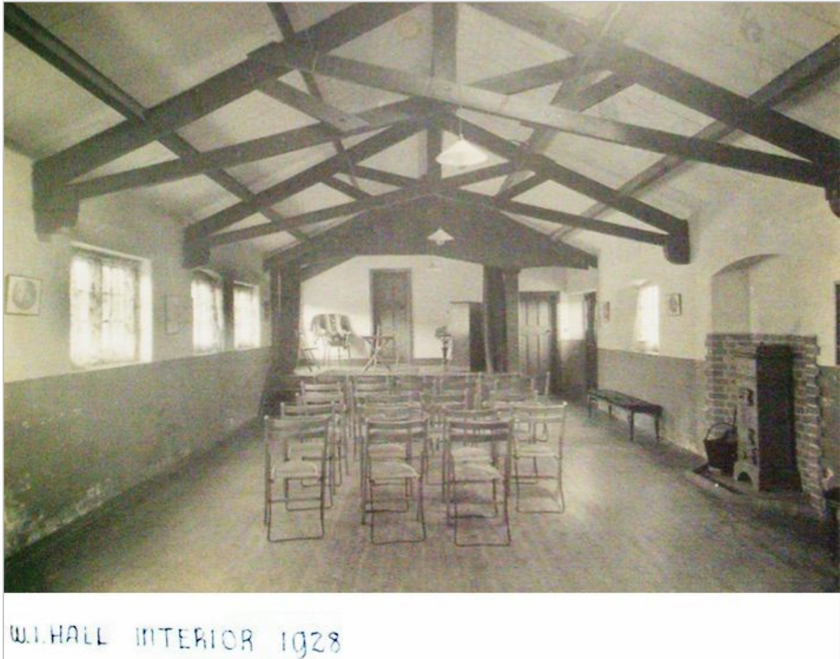
Figure 99 Effingham Women's Institute's new hall, recently completed; photographed in 1928.
