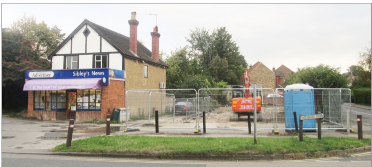
Figure 91 Demolition of the workshop; October 2016.
