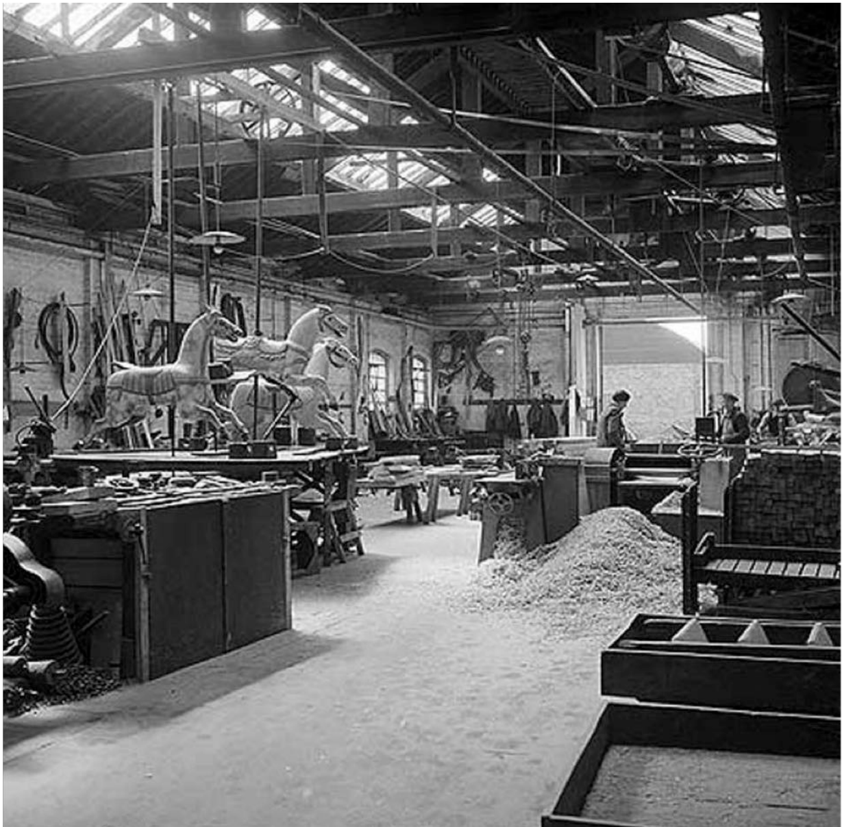
Figure 98 Interior of a workshop at Savage's showing gallopers in preparation.
