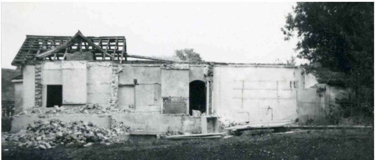
Figure 51 Demolition of the Corner Bungalow in the 1960s.
