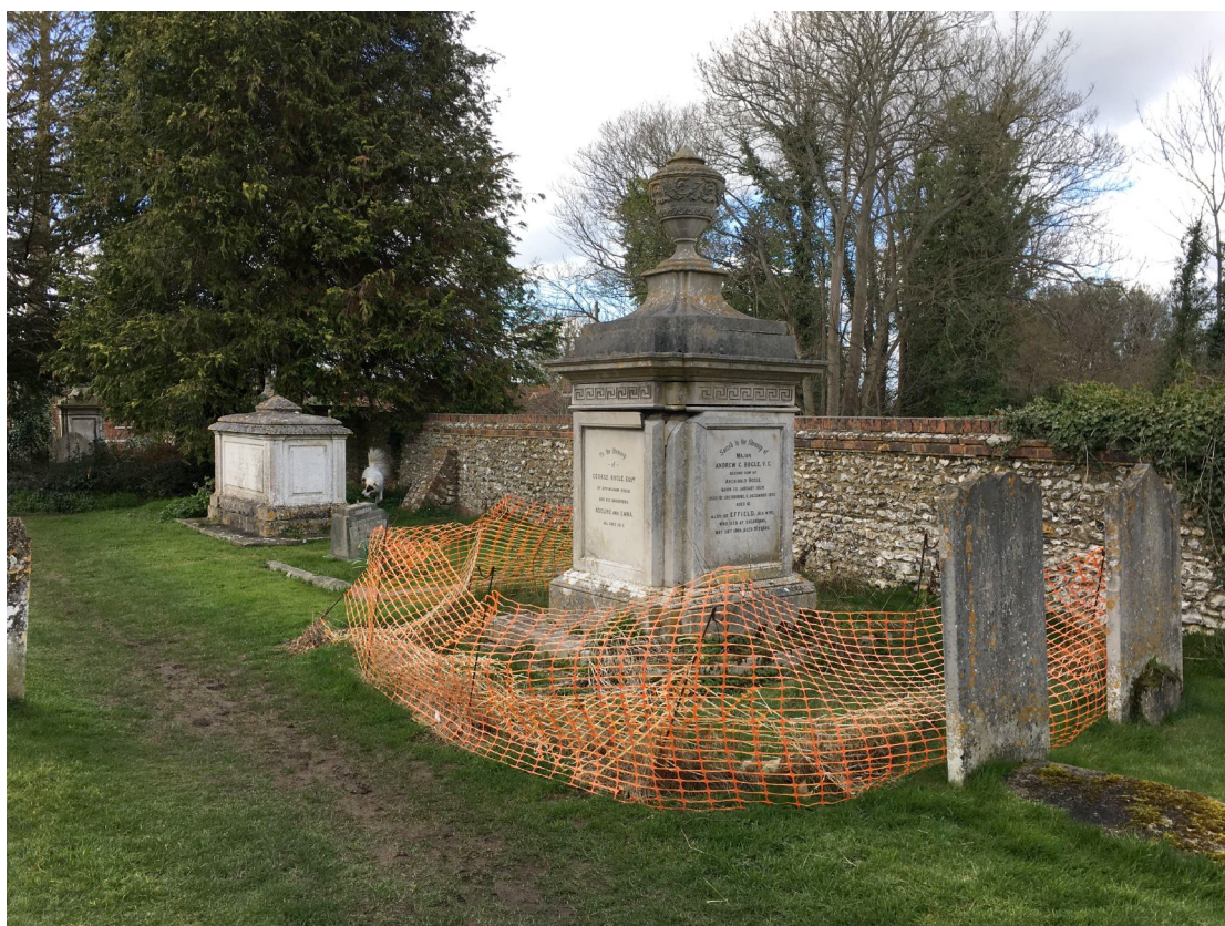
The Bogle tomb in St Lawrence churchyard, currently fenced off because it is unstable. It is nationally Grade II Listed, no 1029427
