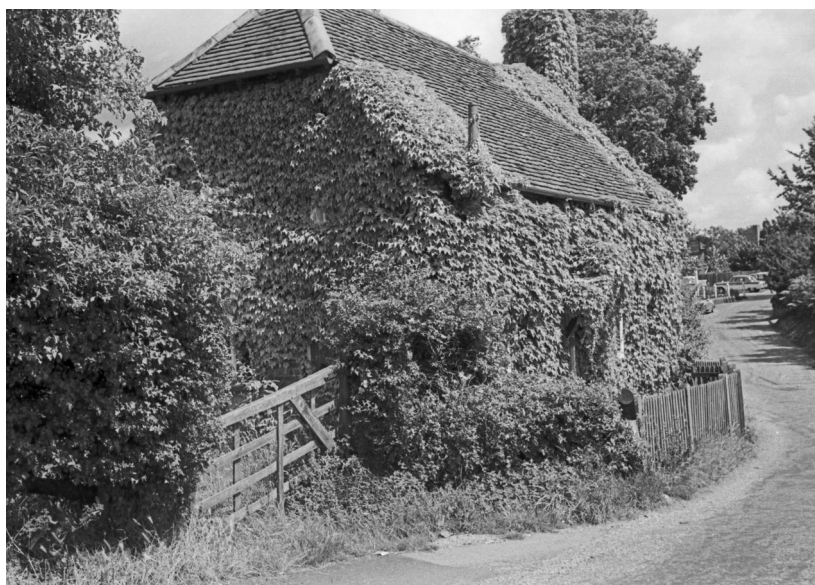
West Lane Farm (Killick's Farm) on Orestan Lane before demolition, early 1960s
