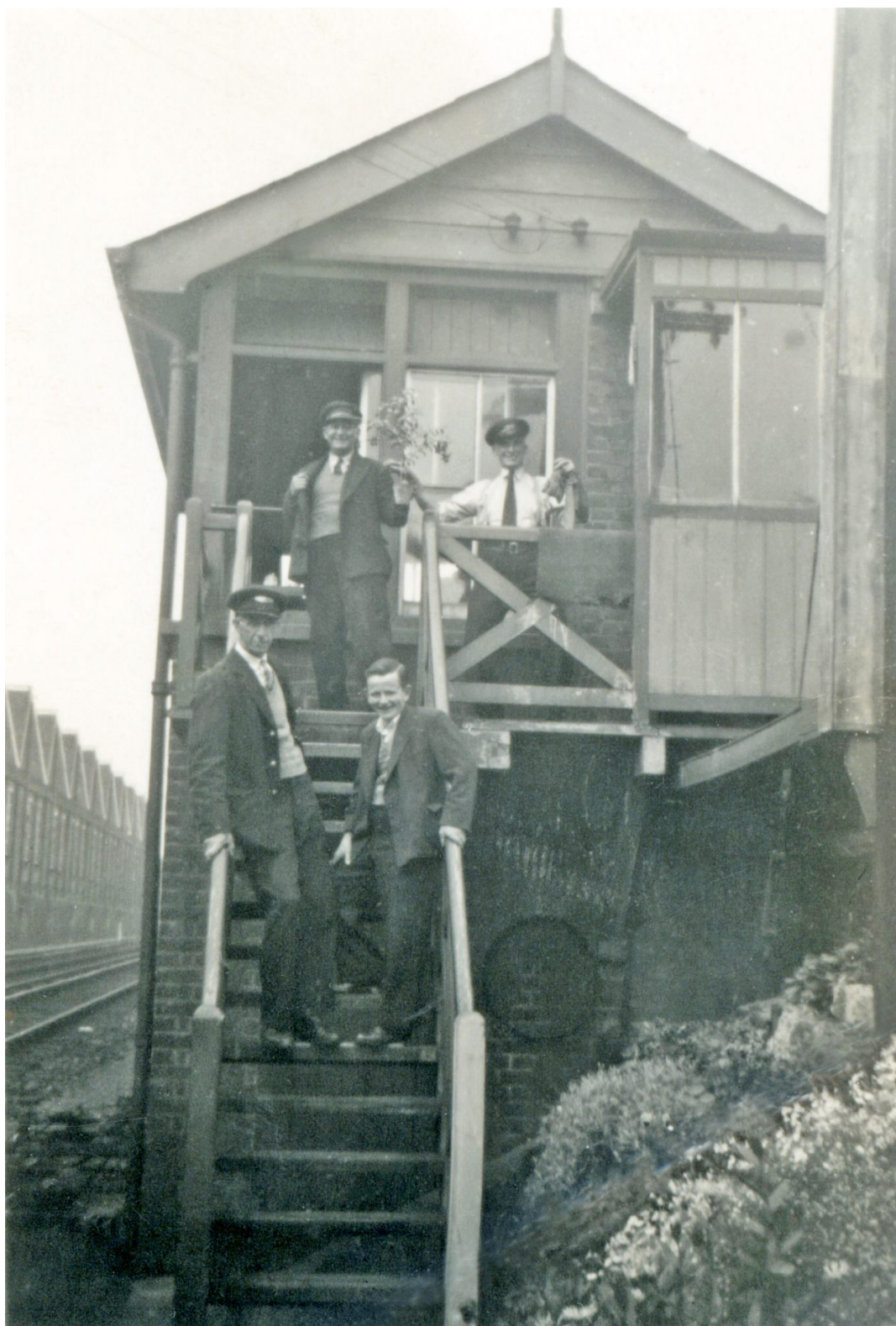
Figure 17 Effingham Junction signal box; Jesse Waller is standing right-most above the steps.
