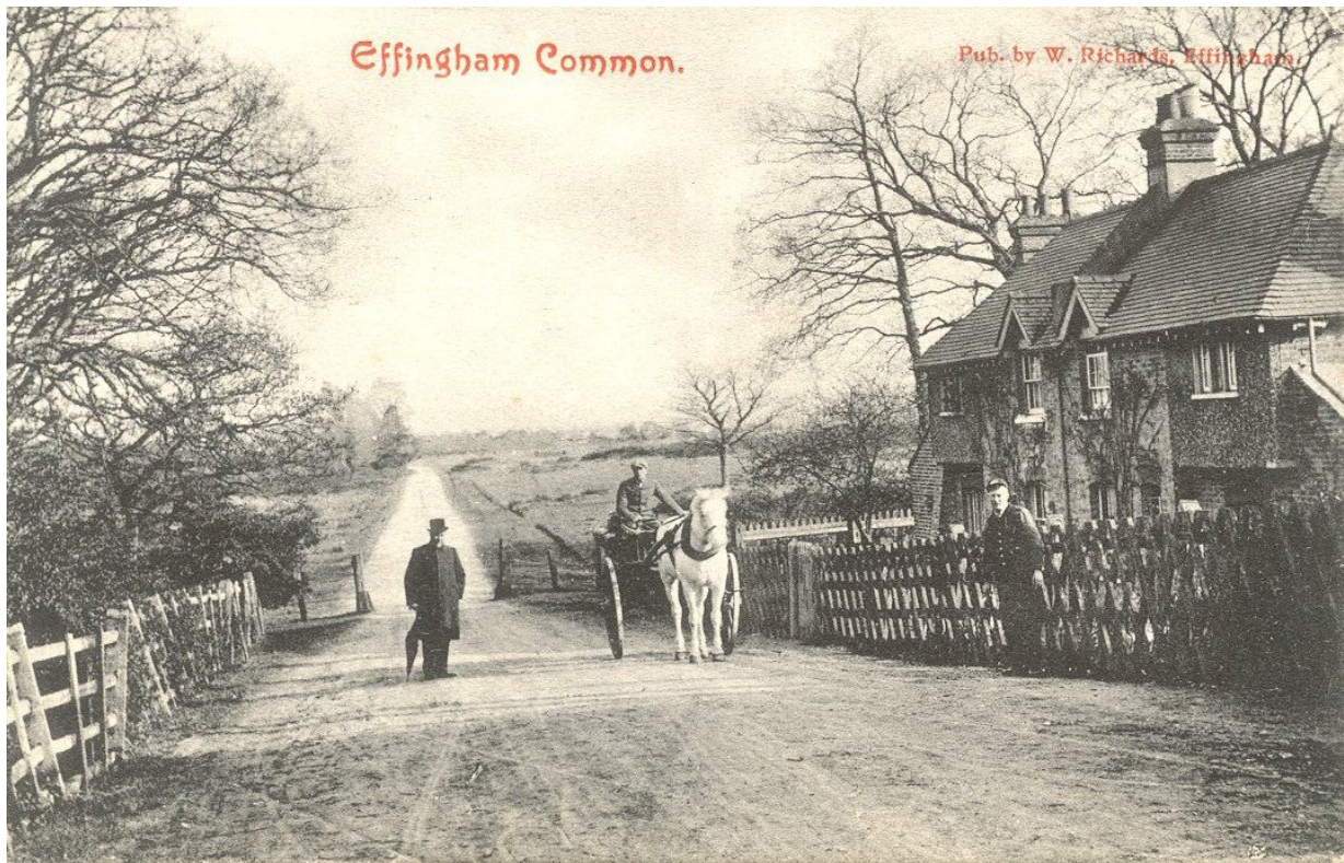
Figure 5 Looking south towards to the Common, with Nos 1 and 2 Station Cottages on the right.
