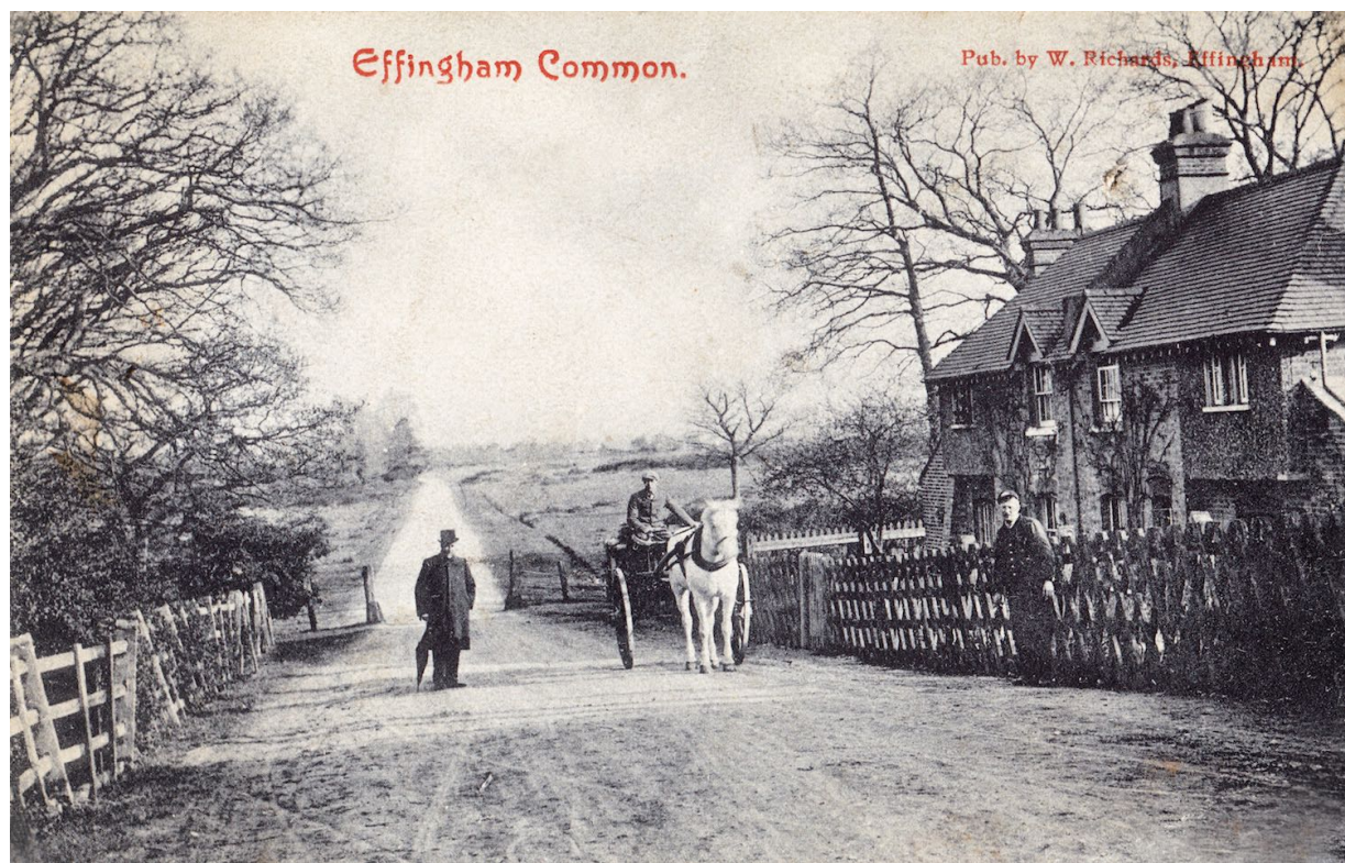
Figure 46 The gate at the north end of Effingham Common; not later than August 1906.
