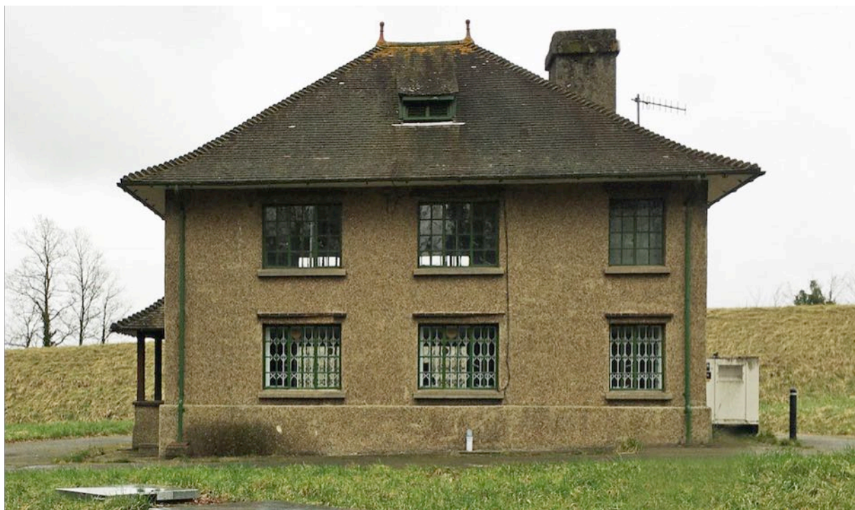
Figure 37 The Beech Avenue pumping station.
