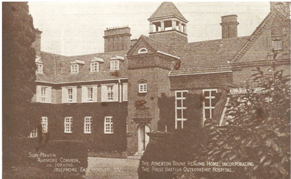
Figure 30 Sun Haven postcard showing the main entrance on the western side of the house, mid-1930s.
