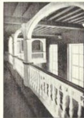
MAIN CORRIDOR TO BEDROOMS
