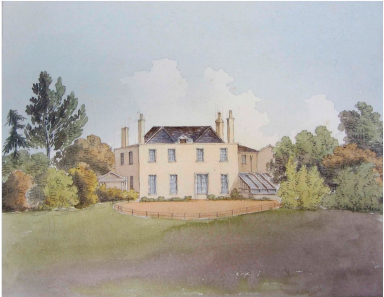
Figure 34 Effingham House in 1823, painted by John Hassell; by courtesy of the Surrey History Centre.
