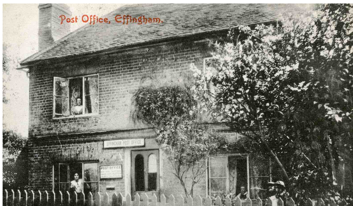
Figure 13 The Butchers at the Post Office (today's Old Post Cottage) in Church Street.
