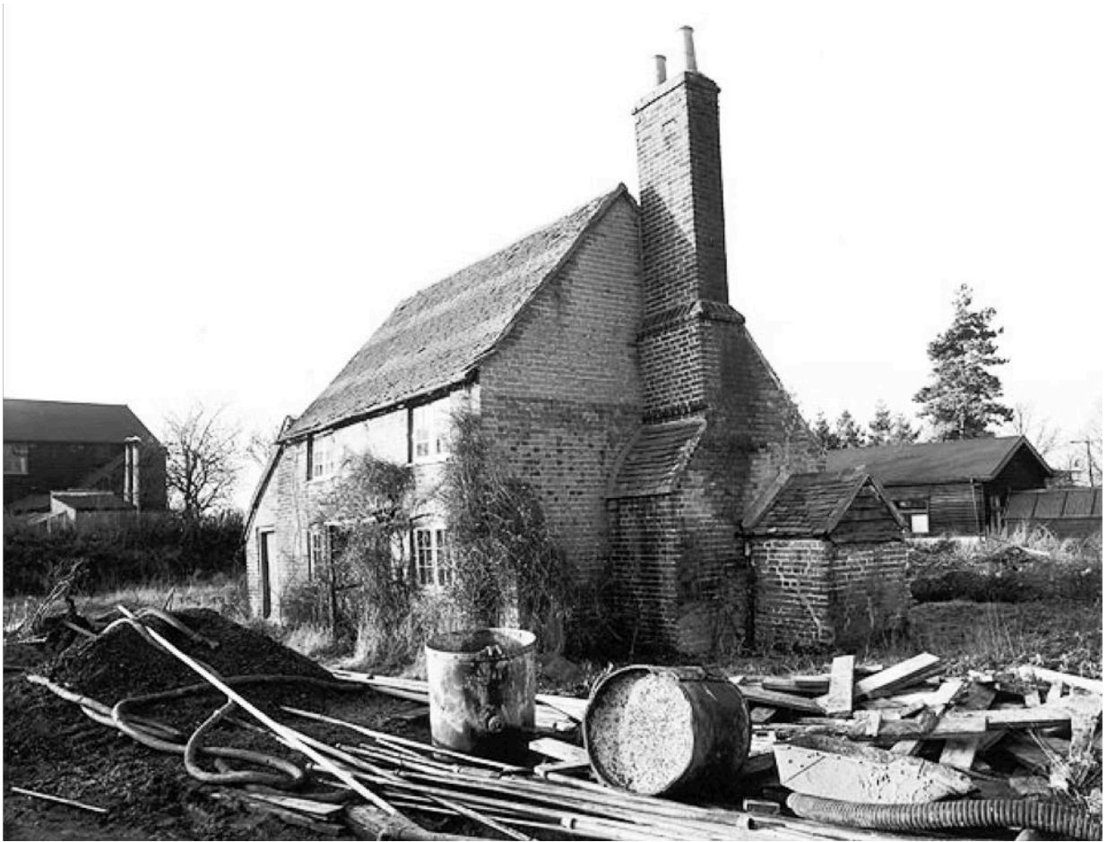
Figure 9 The Lower Road Cottage, looking westwards towards The Red House; at far right is the old hut; 1956.
