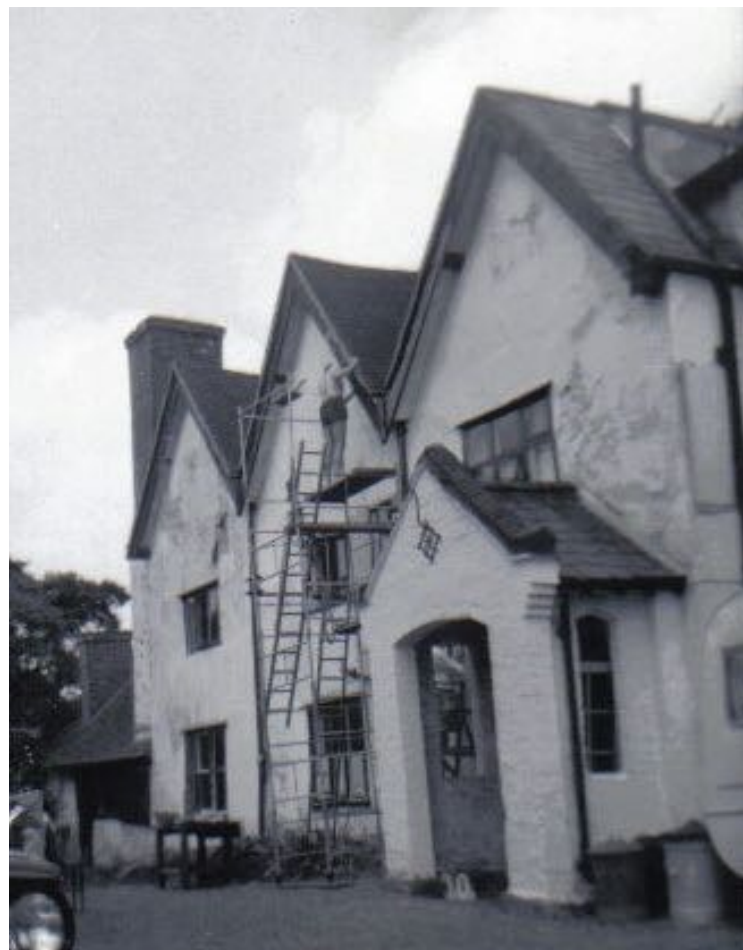
Figure 9 Fitznells in Ewell, under refurbishment in the 1960s.
