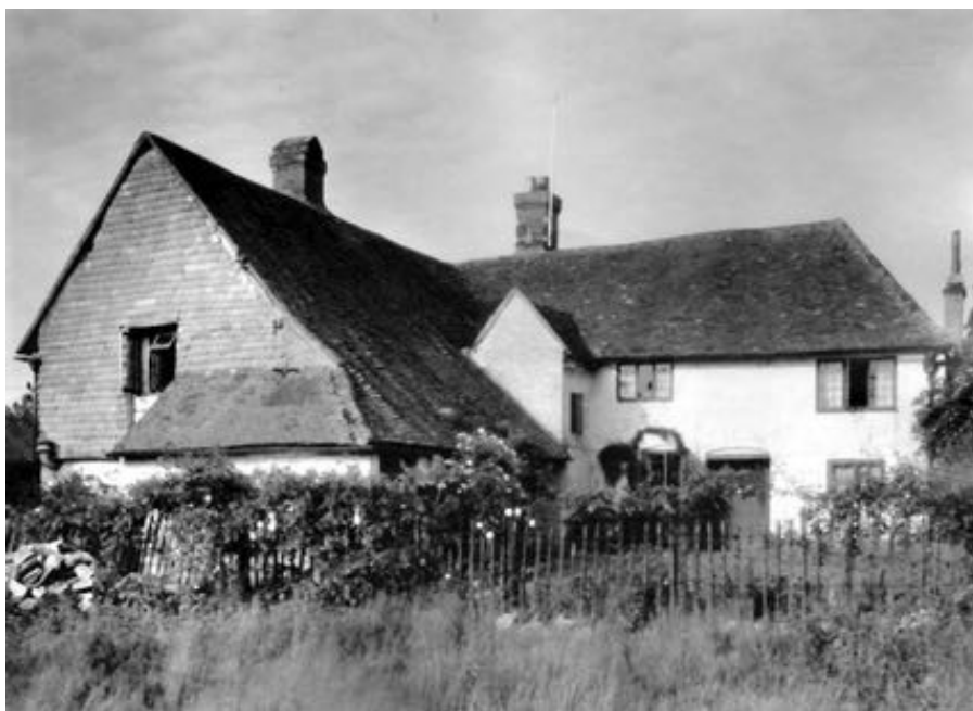
Figure 34 This view of Home Farm appears to be later than the similar view in Figure 26 as some of the brickwork has now been painted white.
