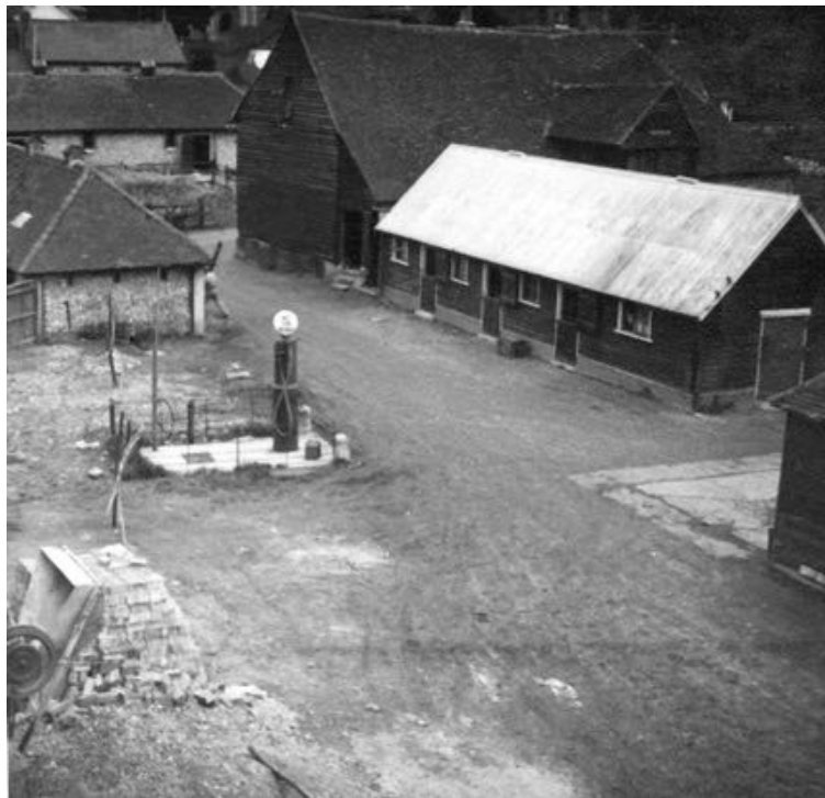
Figure 29 View from the top of the dairy looking SE towards the barn; note the petrol pump.
