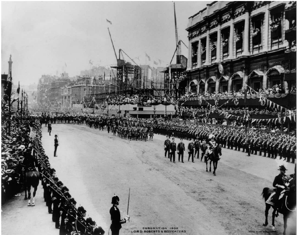
Figure 11 The procession passing the construction site of The Old War Office building in Whitehall.
