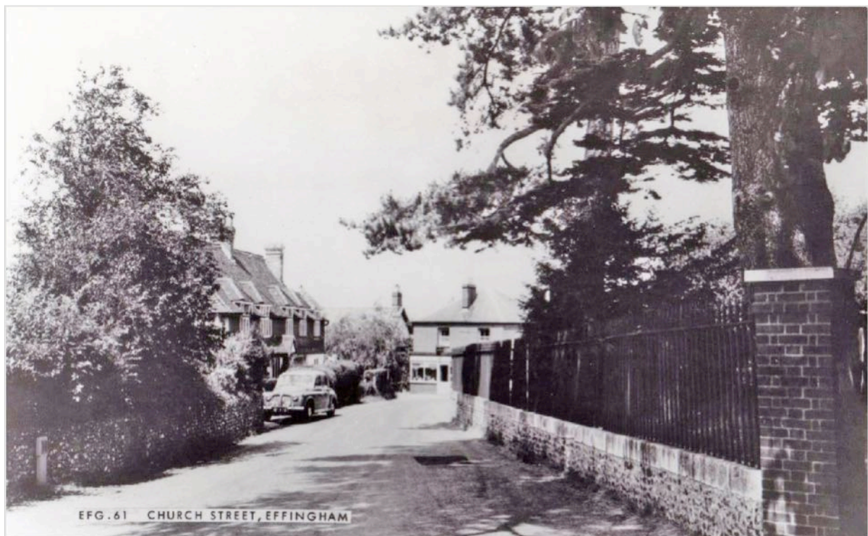
Figure 41 This photograph by Francis Frith appears on an original postcard in the ELHG archives which is neither stamped nor franked and bears no message. However, Frith assigns the date 'c.1965' to it and if that is correct then it shows the stores in Mr Stanton's time.
