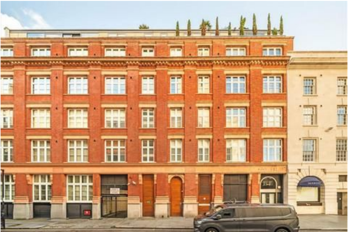
Figure 28 Old Lambert & Butler factory, Wild Street (behind Drury Lane); modern photograph.
