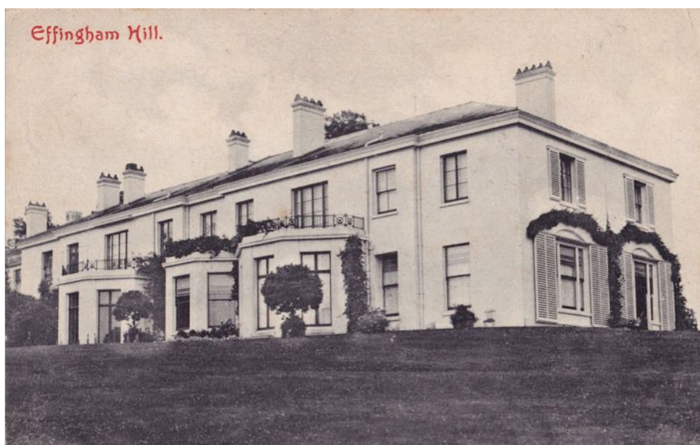
Figure 11 Effingham Hill House, north side; early 20 th C.
